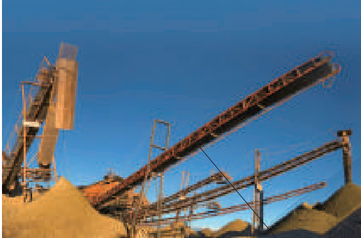
Bulk material conveyors
